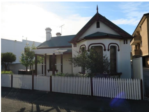
HERITAGE LISTED VICTORIAN DWELLING AT 20 MARION STREET
